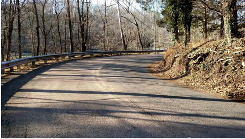
Figure 7 Westbound view of the curve on Headquarters Road located 250 feet east of the intersection with Sheephole Road, the site of 5 crashes within the reporting period
