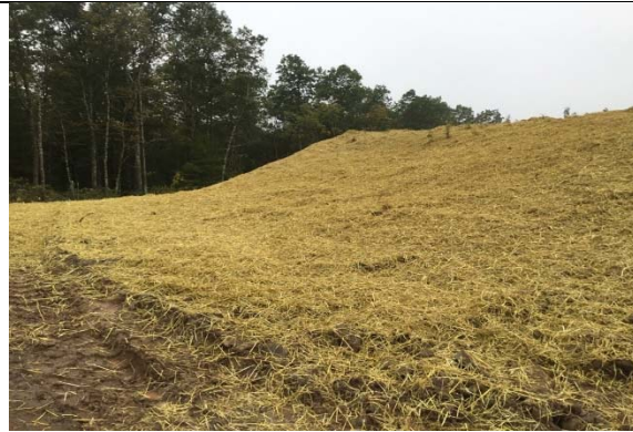
Photograph 2: Area K (Highland) soil stockpile stabilized.
