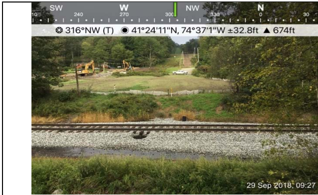
Photograph 1: STA 84+00 (Huguenot) Vegetative where permanent seeding activities have been completed.
