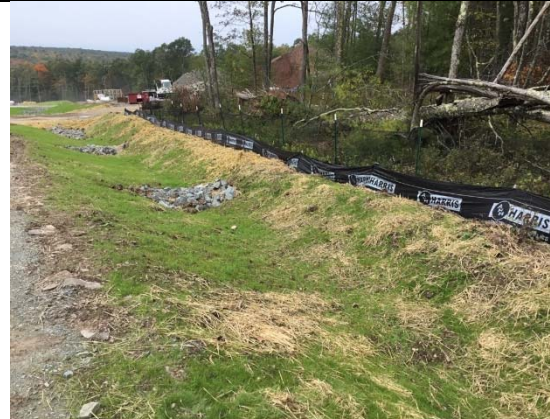
Photograph 4: Area D (Highland) replaced straw mulch and permanent seed mix wash from the edge of the drainage ditch.
