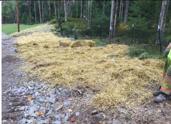
Photograph 3: Area A ROW (Highland) stabilized.
