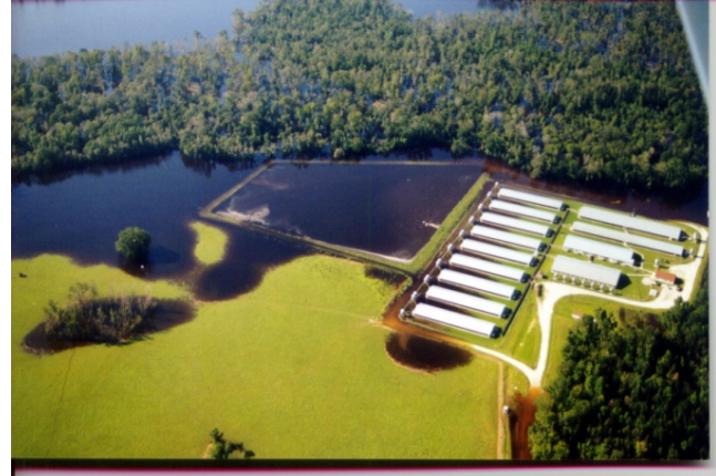
CONFINED ANIMAL FACTORY FARM BEING INUNDATED WITH FLOOD WATERS. THE FARM'S LAGOONS CONTAIN MANURE AND CONTAMINANTS THAT, WHEN FLOODED OR OVERTOPPED, POLLUTE THE NEARBY WATERWAY.
